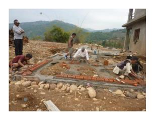
The setting of wall corners to start building female toilet block on 25 April 2015 morning time till 11:30am and
